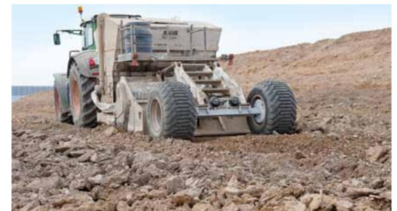
Fendt 930 Vario with a SBF 24-6 soil stabiliser. The mixed binder is determined according to the soil type as well as the moisture class, e.g. B50 is 50% lime and 50% cement (Foto: Daniela Müller)
