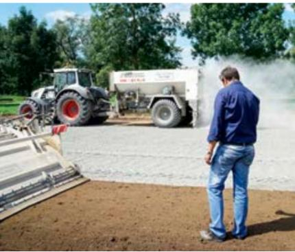
◀ The guidance system is vital to such soil stabilisation work.
