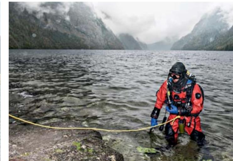
Before transporting the vehicles across the lake, a 3150-metre long, 31-tonne underwater cable was laid down on the ground of the fjord-like lake. Specially trained expert North Sea divers from Hamburg and a team of underwater cable layers from Scotland conducted the work.
